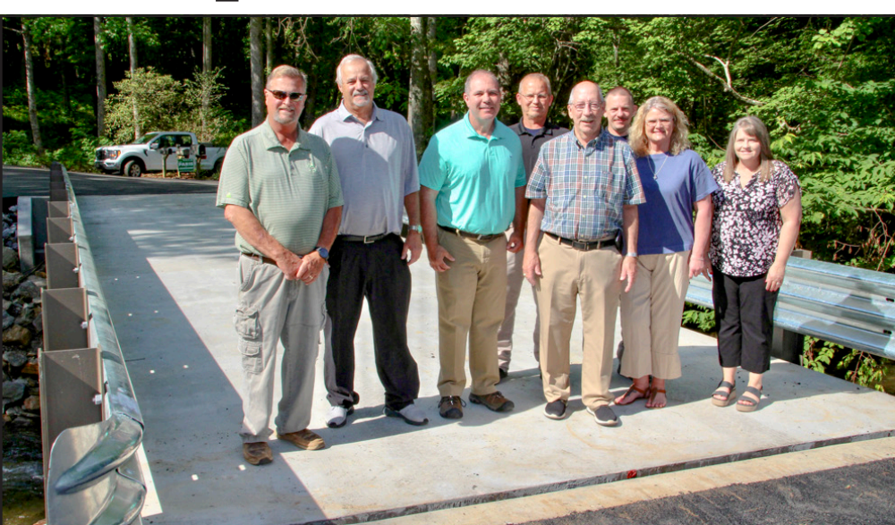
County officials were pleased to open the new permanent bridge over the Nottely River at Fisher Field Road last Wednesday. Photo by Shawn Jarrard
